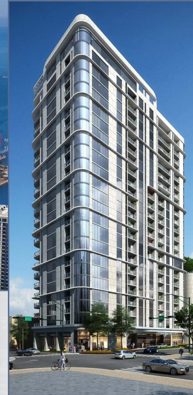
Onyx Apartments UNDER DEVELOPMENT 224 units 22 story luxury apartment tower
