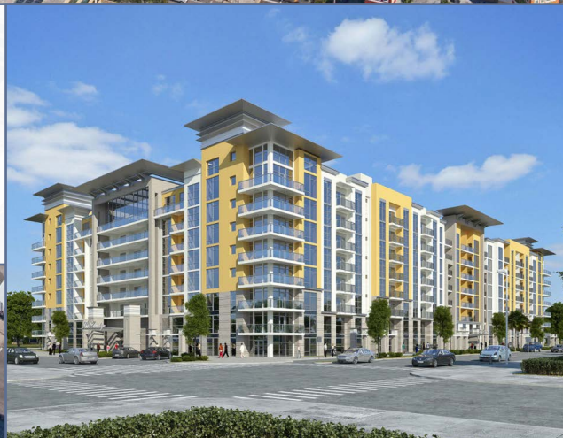
The Heritage COMPLETED $65 MM project 8 stories 348 apartments
